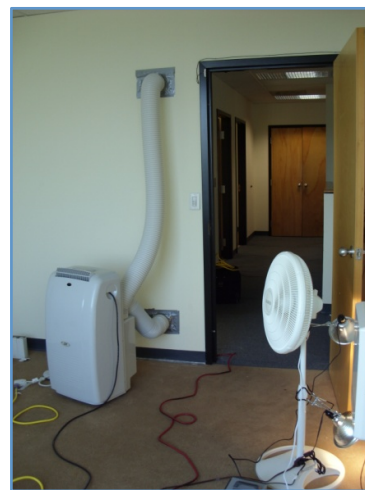
Figure 5. Cooling Unit, Mixing Fan, and Variable Light Loads
